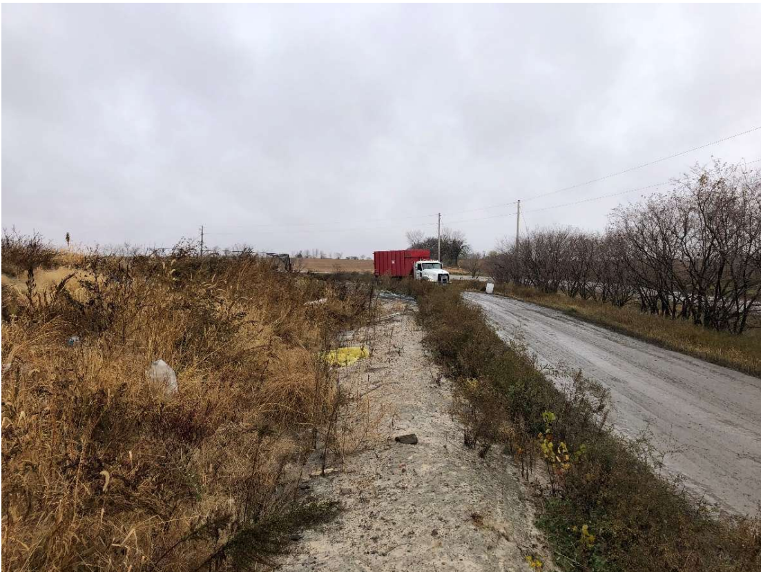
Photo 30: Location 11 – Looking North, Phase 4 Eastern Anchor Trench
