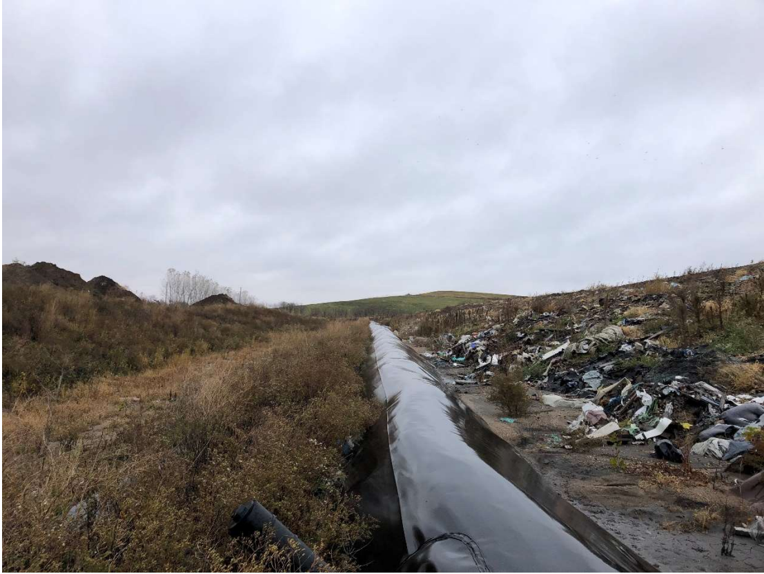
Location 13 – Looking East, Phase 4 Northern Rain Flap
