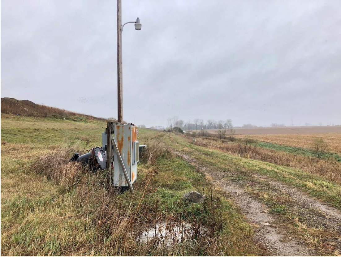
Location 6 – Looking East, Phase 2 Southern Slope
