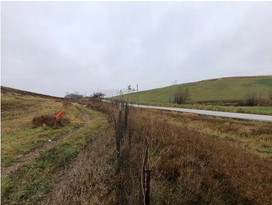
Location 8 – Looking North, Phase Eastern Berm
