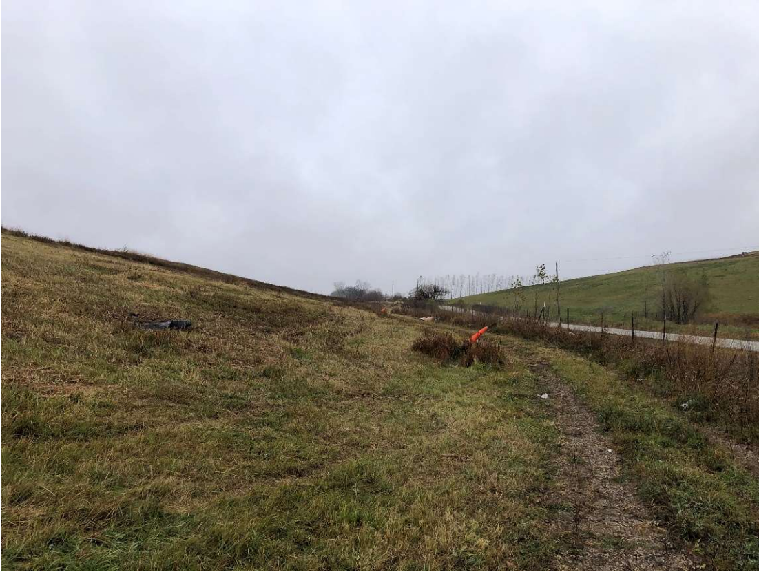
Location 8 – Looking North, Phase 2 Eastern Slope
