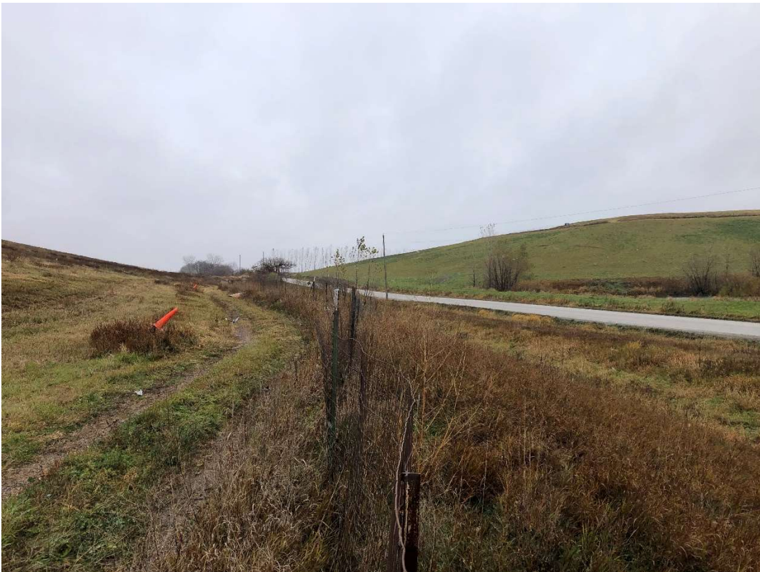
Location 9 – Looking North, Phase 2 Eastern Berm
