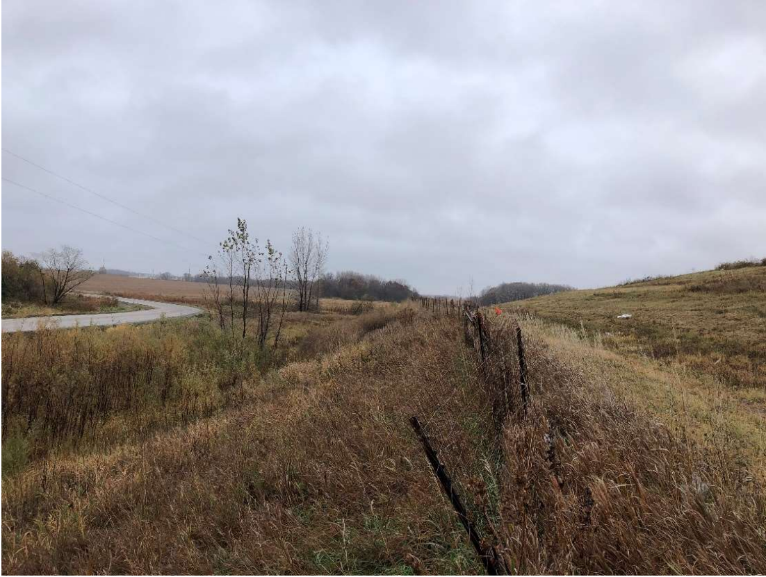
Location 9 – Looking South, Phase 2 Eastern Berm
