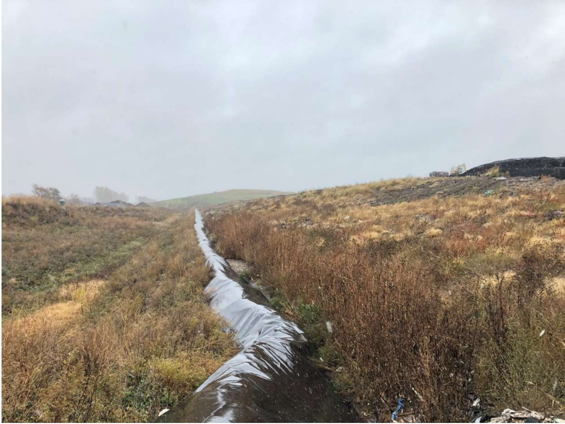
Location 1 – Looking East, Phase 4 Northern Rain Flap
