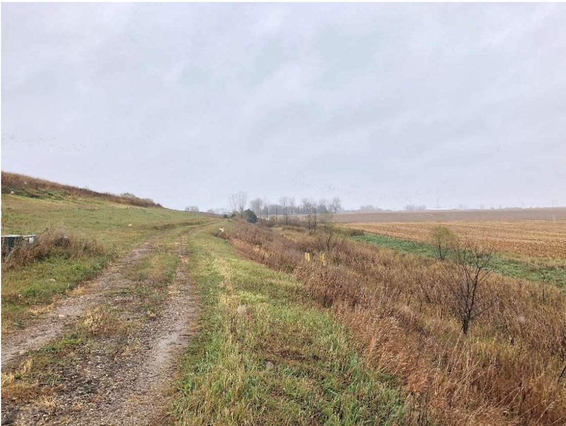
Photo 14: Location 6 – Looking East, Phase 2 Southern Berm
