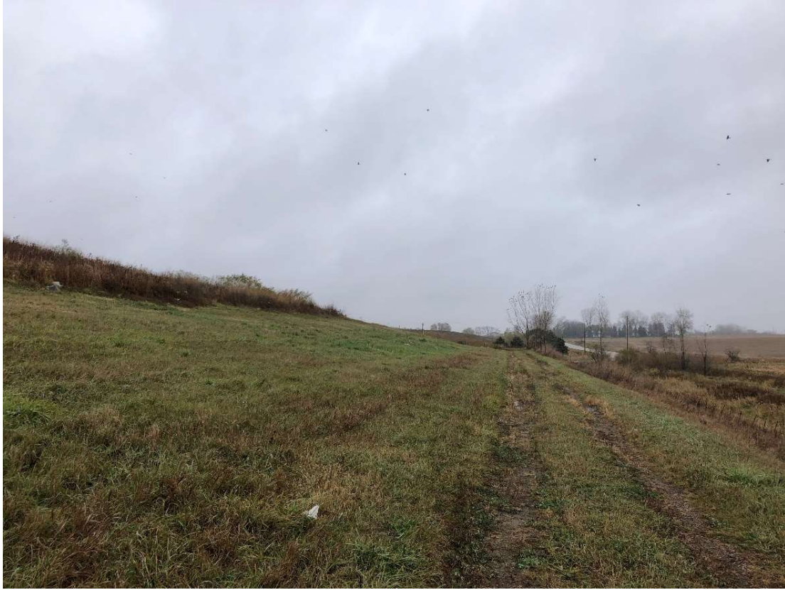
Location 7 – Looking East, Phase 2 Southern Perimeter Road and Slope
