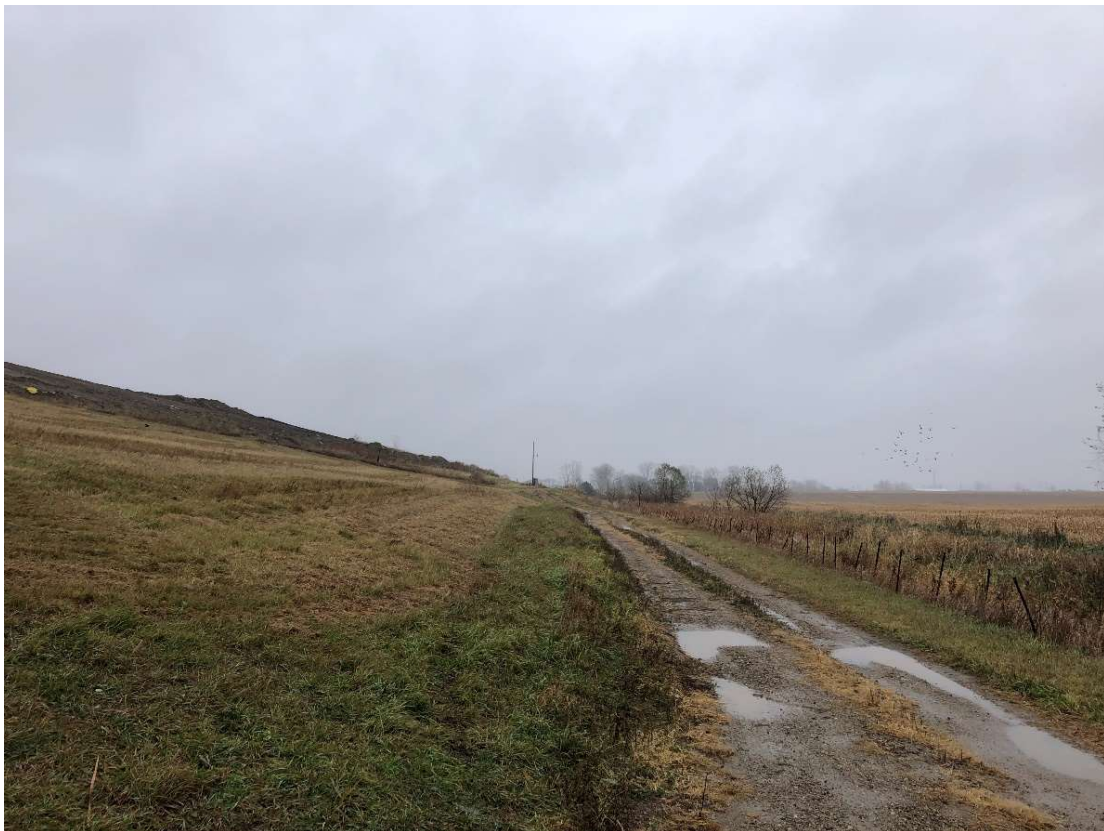
Location 4 – Looking East, Toe of Phase 1 Southern Slope
