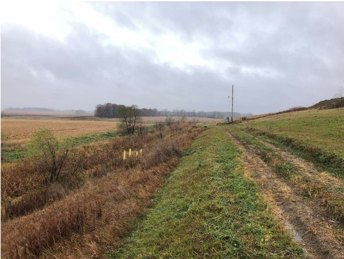
Location 7 – Looking West, Phase 2 Southern Berm
