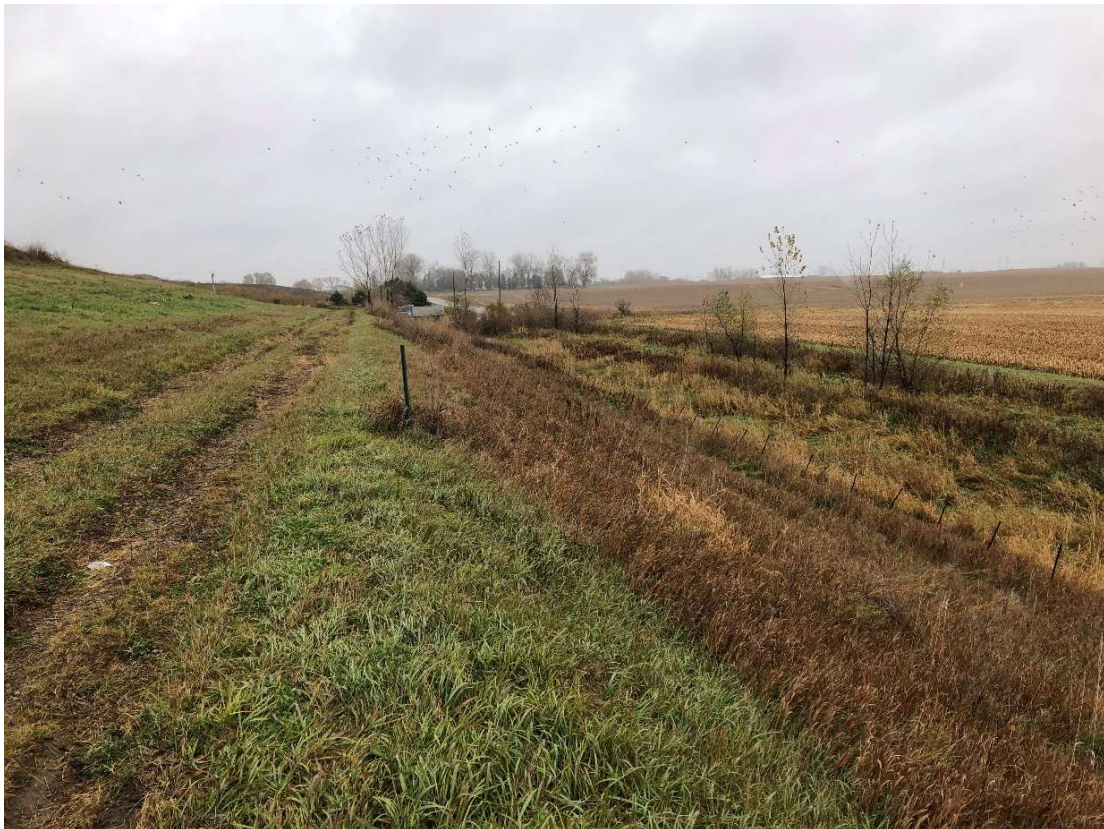
Location 7 – Looking East, Phase 2 Southern Berm
