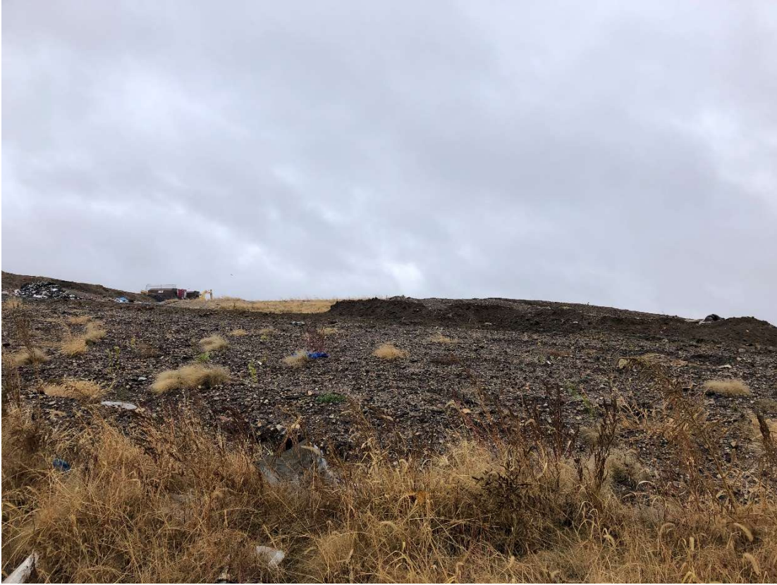
Location 11 – Looking West, Phase 3/4 Connection, Phase 3 Norther Interior Waste Slope
